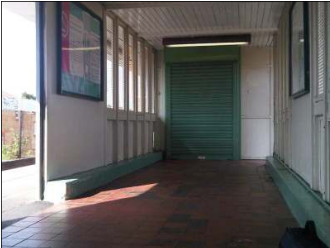
(12) Booking office window (closed and shuttered, unstaffed), seen from the staircase, 16/9/09
