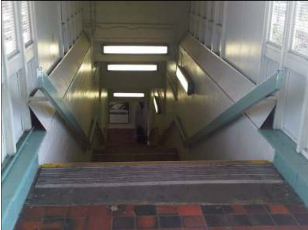
(11) Staircase seen from platform level, 16/9/09
