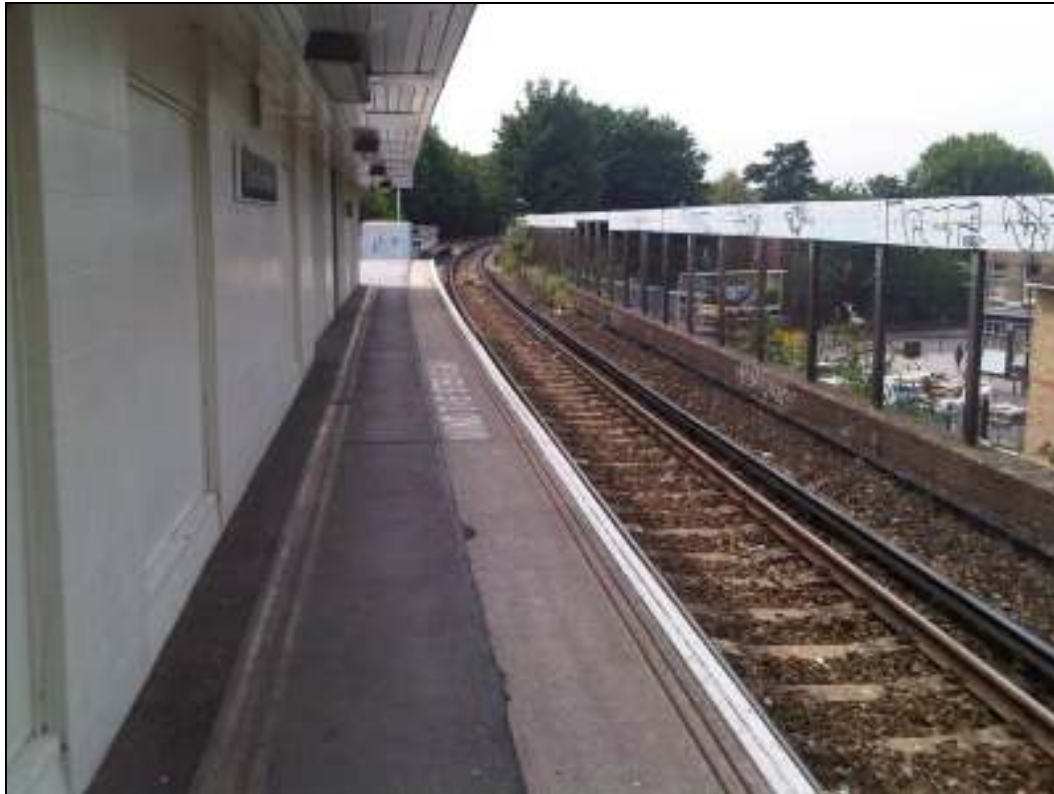
(17) Platform view southbound towards Peckham Rye, also showing the trackside fencing, 6/8/09
