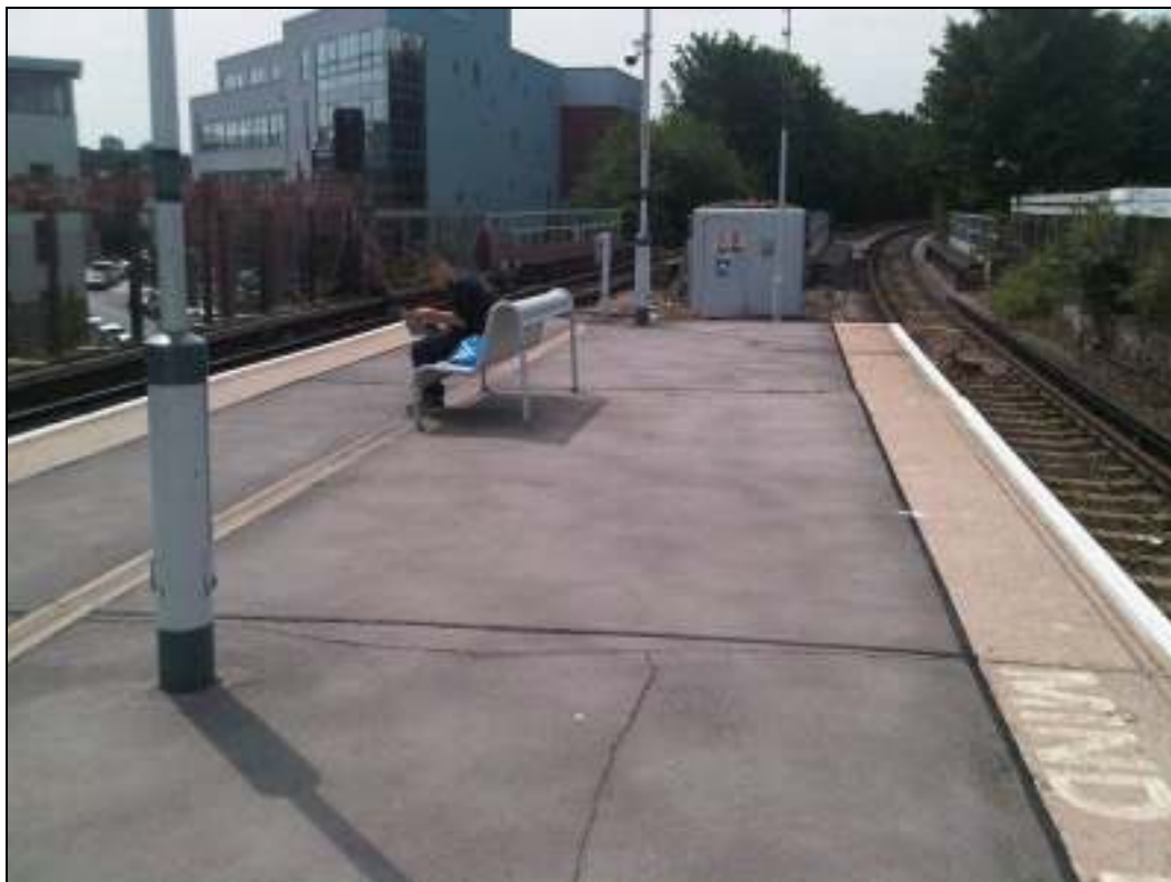
(18) Southern end of island platform looking over Queens Road, 6/8/09. Ultimately a passenger lift might be located south of the platform, between the two rail bridges with the hut relocated (see JRC proposals)
