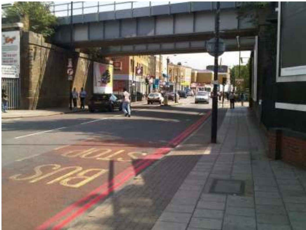
(4) View east at Queens Road Peckham, 6/8/09, under the railway bridge towards the station, with the National Rail sign only just visible from the westbound bus stop. The eastbound bus stop is in the distance
